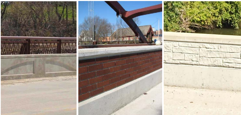
Figure 5.8.1.2.5-4. Examples of Barrier Traffic Face Treatments
